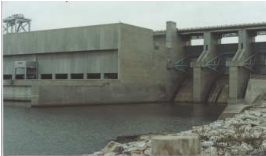
Figure 1. Example of a steel-reinforced concrete dam.
