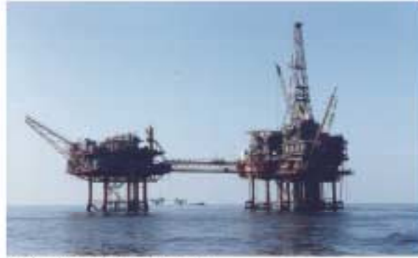
Offshore oil drilling platform
