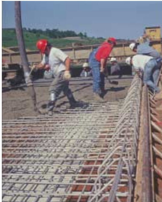
Figure 14. Stainless steel-clad rebar deck construction.
