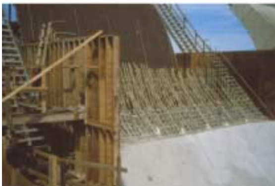
ALSEA bridge, Oregon, with epoxy-coated rebar substructure
