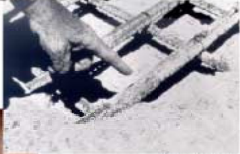
Corroded rebar
