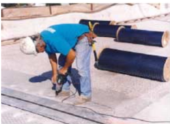
Installation of titanium mesh impressed-current anode system on bridge deck
