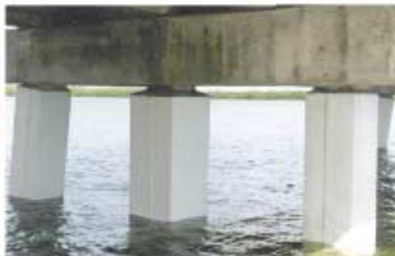
Sacrificial CP applied to pier columns in marine environment
