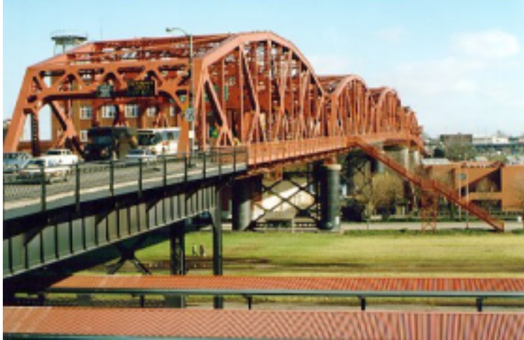
Figure 3. Steel bridge structure.
