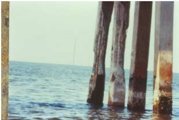
Figure 10. Examples of substructure corrosion.
