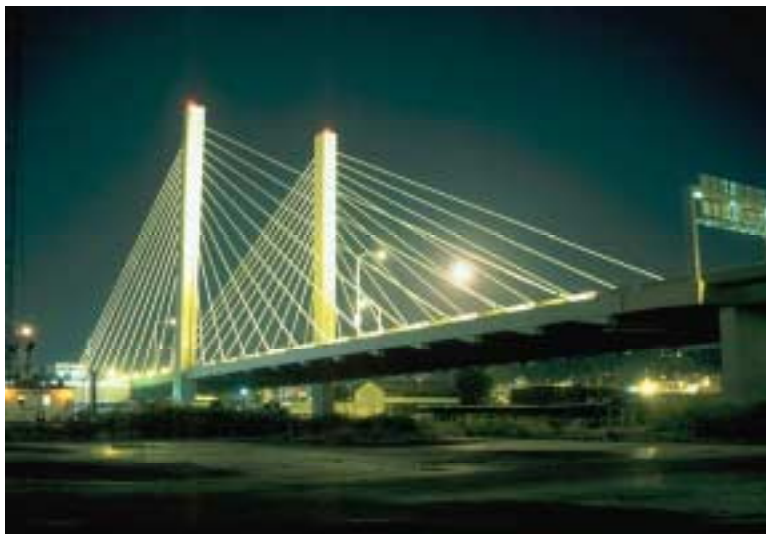
Figure 6. SR509 bridge in Tacoma, WA (cable-stayed).
