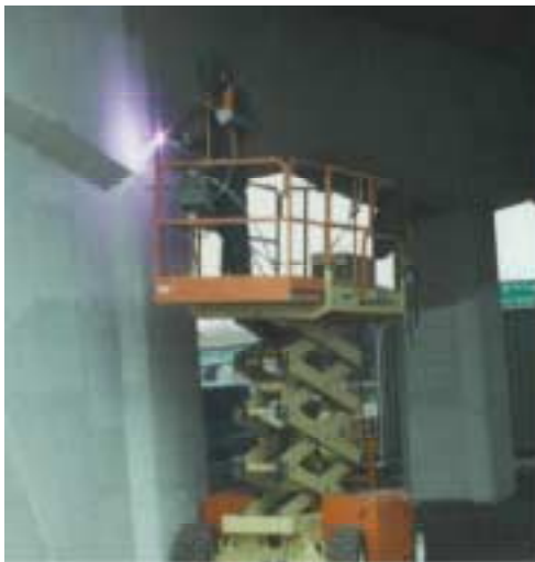
Application of thermal spray metal coating as sacrificial anode system on bridge pier
