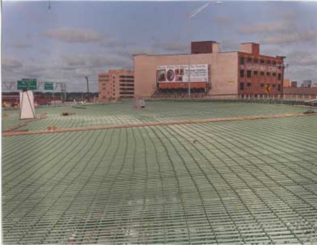
Figure 13. Epoxy-coated rebar deck construction.
