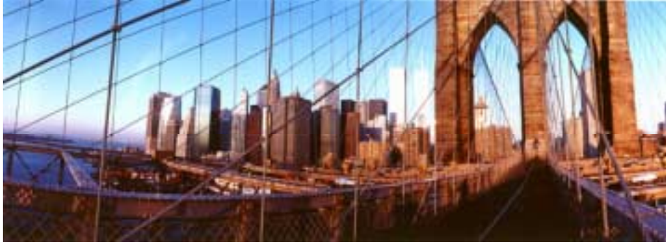
Figure 5. Brooklyn Bridge (suspension).
