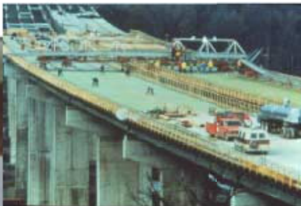
Epoxy-coated rebar construction on deck
