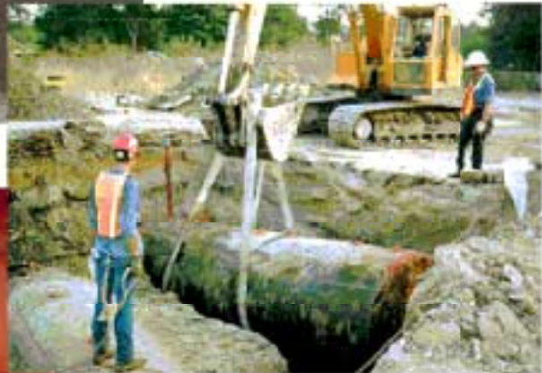
Lifting underground storage tank
