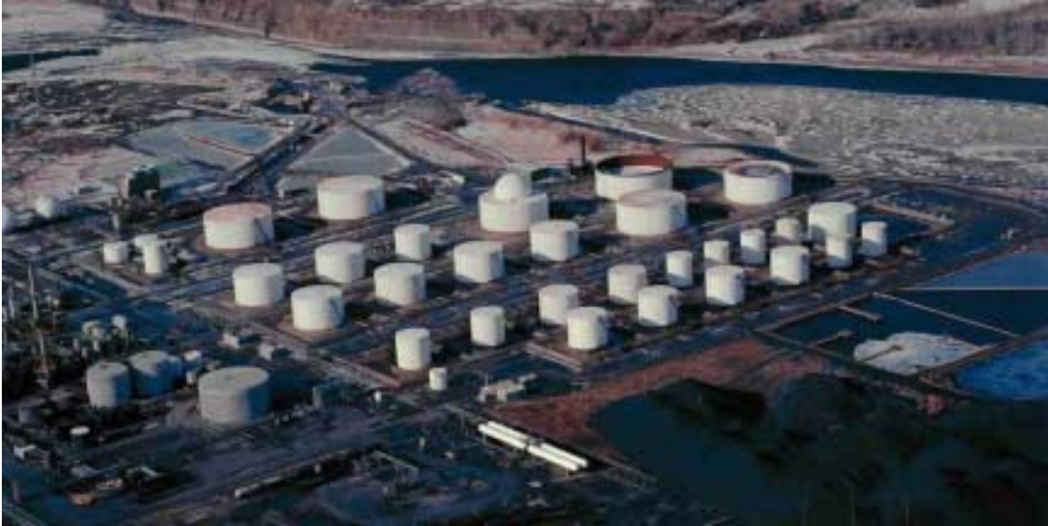
Figure 2. Example of an oil storage tank farm, showing multiple tanks of varying sizes.
