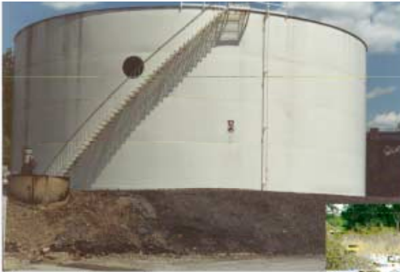
Aboveground storage tank
