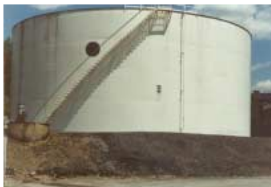
Figure 1b. Unpressurized storage tank.
