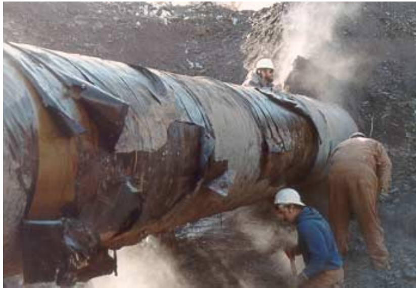
Figure 9. Inspection dig and pipeline repair.
