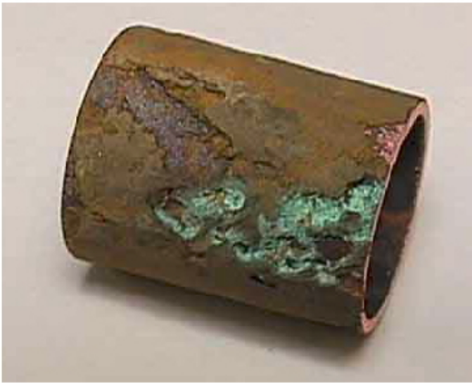
Piece of gas pipeline with external corrosion
