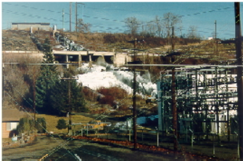
Frozen water from leaking cooling water supply line
