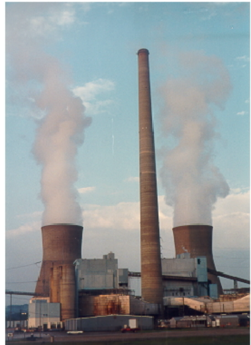
Stack and two cooling towers
